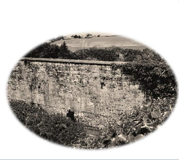
THIS WAS ACHIEVED BY MAKING A WALL HOLLOW, SO THAT A FIRE COULD BE LIT, WITH OPENINGS ON THE GARDEN-SIDE TO DIRECT THE HEAT TOWARDS THE PLANTS, AND A FLUE AT THE TOP FOR THE SMOKE.
