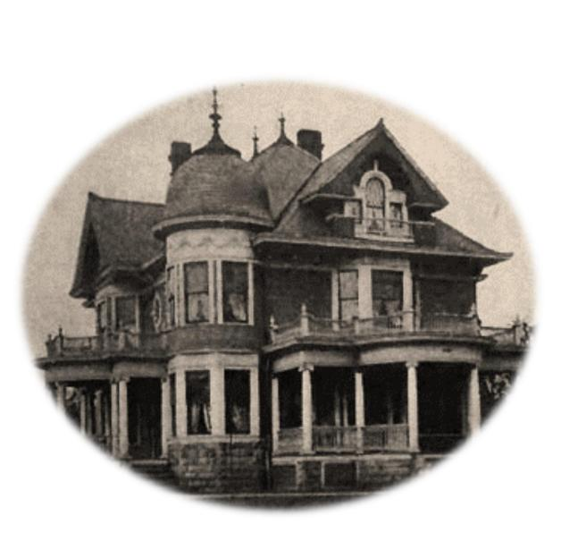
WITH THE ADVENT OF NAILING 2X4 BOARDS TOGETHER (FRAME CONSTRUCTION) INSTEAD OF USING HEAVY TIMBERS, THE FINISHED HOME WAS NOT AS HEAVY... THUS, CREATIVITY COULD RUN RAMPANT.
